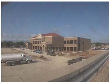
Construction nears completion for the new Abilene Regional Campus.
